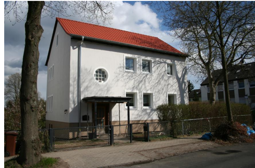
After reconstruction according to passive house principle
